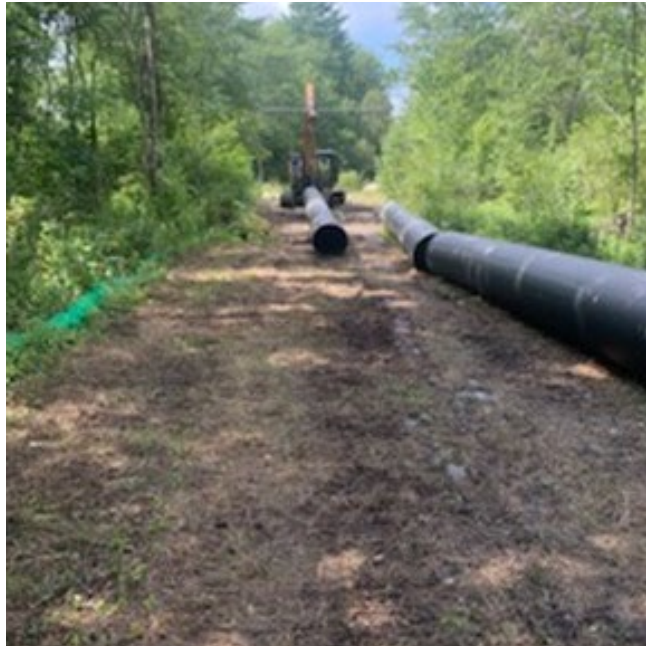
Photo 1: Staging of 20-inch HDPE Sewer Force Main in Cross Country Easement
