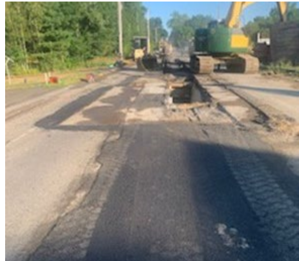
Photo 3: Installation of 20-Inch PVC Sewer Force Main on Auburn Street
